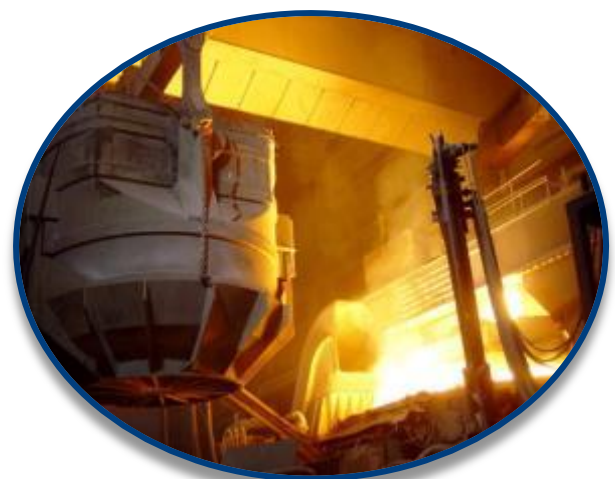
Electric Arc Furnace
